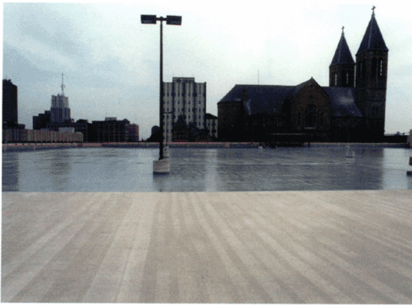
A polyurethane-based traffic-bearing deck coating applied across the entire top level of the University of Akron's refurbished parking garage adds watertight and non-skid properties to the concrete. Compatible with the nosing material that adhered the Santoprene rubber expansion joints to the concrete, the deck coating ensured continuity between the seal and the deck expansion joint system.
