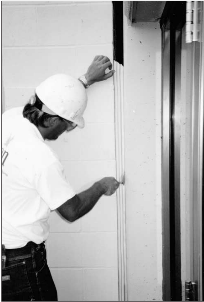
Hybrid silicone/impregnated foam sealant is inserted into joint-gap.
