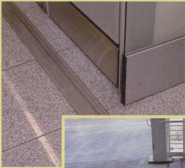
Interior joints are aesthetically versatile and offer a lasting alternative to "rubber and rail" joints in high-point load stadium environments.
