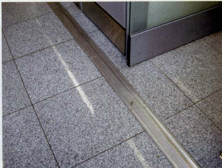
Interior joints in high-point load stadium environment
