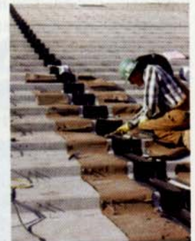
Factory-welded, custom tread and riser joint systems ensure durability and watertightness
