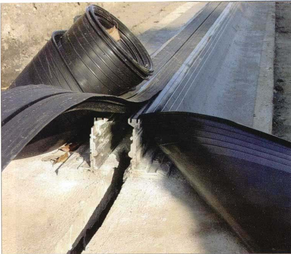
Migutan system components—retainer legs installed onto structural slab, side flashing sheets, and movement gland—before installation of stainless steel retaining caps and before integration into the deck waterproofing membrane.
