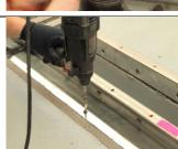
**Vacuum** dust piles from around holes. **Blow** dust from inside the holes using a forced-air blast and then **vacuum** again.
