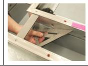
Continue the above process along the entire length of the expansion joint system. Check length of final piece(s) and mark for cutting.
