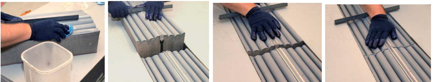
16) If the spline pin did not seat all the way in step 15, use a 3-pound hammer to tap the aluminum part of the end of the spline away from the joint to ensure that the spline-pin is driven all the way into the previously installed length. (Note: liquid silicone should squeeze up out of the joint).
