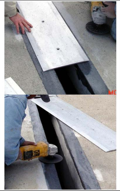
**6) Mix one kit of epoxy adhesive and apply a thin coat (no more than 1/16" thick) to both joint faces to a depth of 4-inches (100mm)—be sure to extend epoxy between parapet or split column faces of transitions to upturns.****Mixing Epoxy:**
