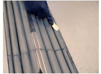
23) Starting at one end of the joint, remove the first one or two hangers to make room to install the first section of coverplate.
