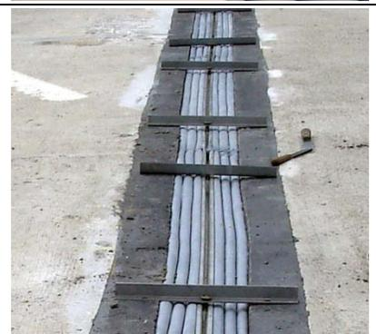
19) Using lint-free cotton rags and solvent clean the silicone bellows next to the joint faces to receive the silicone sealant bands and corner beads.
