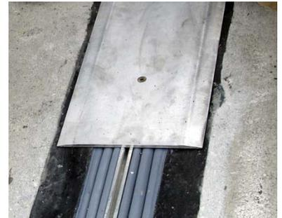
26) Using a drill-driver and 7/32" hex bit socket, drive the coverplate screws into the spline channel until tight. Ensure that the spline is drawn up snugly against the underside of the coverplate. If necessary, use a hand socket wrench and handle extension to do the final tightening.
