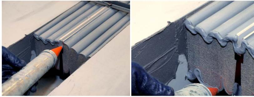
13) Using a large (20 ounce) bulk caulk gun and the intumescent caulk sausage provided, gun intumescent caulk on the foam face of the end of the material.
