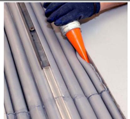
22) Using a caulk knife, tool the silicone into a corner bead between the top of the silicone bellows and the joint face.
