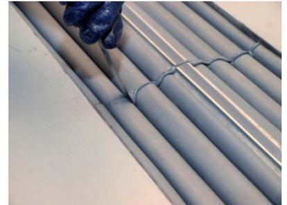
18) Repeat process until all lengths of joint assembly have been installed.
