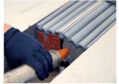
14) Using a caulk knife, spread the intumescent across the foam and spline face to an even 1/8" (3mm) coating.
