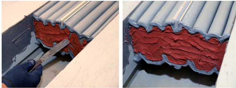
15) Unpack and wipe next material assembly, and lower it into the joint against the wet epoxy on the joint faces, sliding it up to align with the already installed piece.
