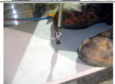
27) Remove next hanger bar(s) as needed and install coverplate sections until installation is complete with the installation of the final finishing cover plate.
