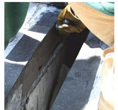
**7) Prepare a "starter piece" of SJS-FR, to suit the transition or termination detail suitable to the joint as agreed in discussion with EMSEAL and EMSEAL field technician.**
