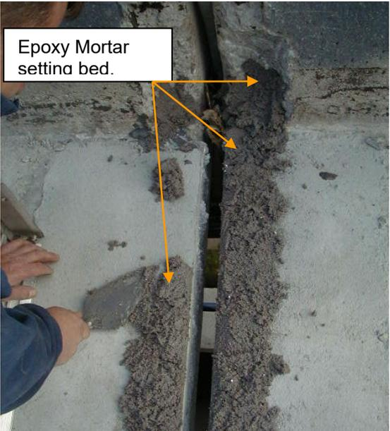
Epoxy Mortar setting bed.
