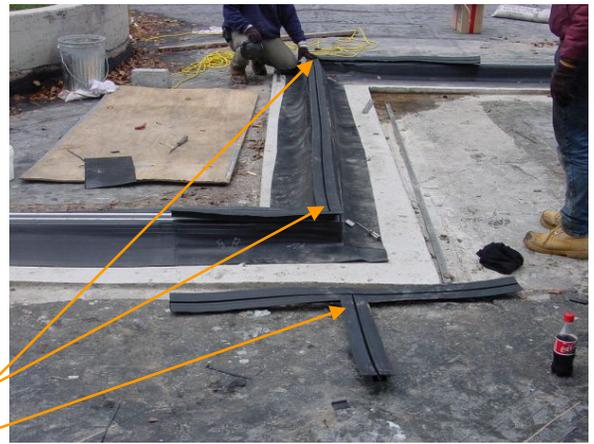
**SPECIAL CONDITIONS:****ANCHORING THE FP.../25 with side-sheets and counter sunk anchors**
