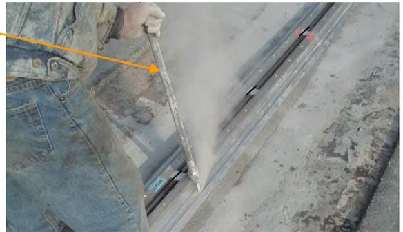
**STEP 9: Install Epoxy Anchors**
