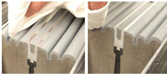
Prior to installation, this release agent must be wiped off all surfaces that will later make contact with liquid applied silicone. This includes, the face, tops and grooves of the bellows next to the face, and along the sides.
