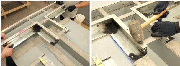
Working away from the ends of the transition, connect the straight lengths of rail and install straight lengths.
