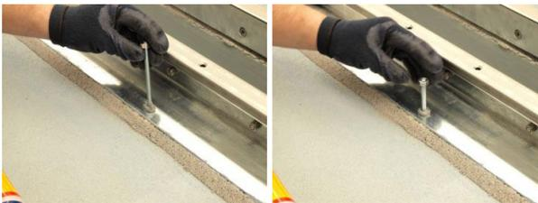
Remove excess epoxy from around the nut that might obstruct tightening later. Allow epoxy to cure according to chart(s) on epoxy cartridge.
