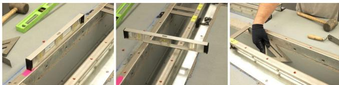
Using a margin trowel remove epoxy that squeezed out from under the mounting flanges into the joint. Use the extra material to pack and fill in voids under the mounting flanges.
