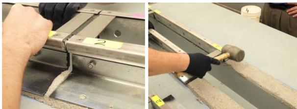
Repeat procedure until final section is reached. Install final section by lifting previous section slightly until the sections can be interlocked. Ensure that all sections are level along and across the joint and that the joint faces align with the faces of the FP legs.
