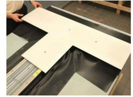
**NOTE** – The screws are self-tapped into the spline anywhere along the spline. You do not have to align the plate holes with the holes where the hanger-bars were attached.
