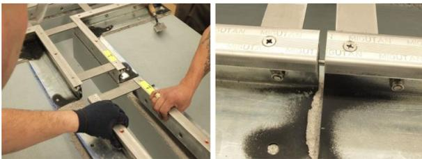
Ensure that joints are properly executed to achieve proper appearance and performance. There should be no gaps between adjoining capping strips.
