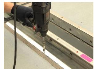
**NOTE** – If obstructions or other conditions prevent full depth embedment, drill holes as appropriate ensuring that anchor-bolts embed at least 3-inches (75mm) into concrete. For depths less than 3-inches (75mm), consult EMSEAL. Vacuum dust piles from around holes. Blow dust from inside the holes using a forced-air blast and then vacuum again.
