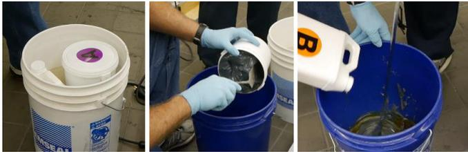
Immediately add the sand from the original EMSEAL pail into the A+B mixture. Pour into center of the mixture, while stirring with the heavy-duty mixing drill and 3-inch diameter mixing paddle. Blend the epoxy and sand to a uniform gray color and consistency (approx. 2 minutes after sand is fully added).
