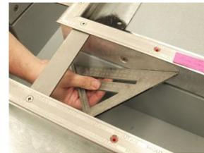
*IMPORTANT: In order to perform as a fire barrier, the SJS-FP-FR foam assembly must install into concrete below the metal FP legs. For this to happen, the faces of the mounting rail legs must be flush to the concrete faces of the joint opening.*
