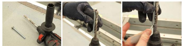
Drill 3/8-inch diameter holes for the 5/16-inch diameter anchors (or as otherwise specified for the particular job or anchoring system — consult EMSEAL). Drill holes to a depth to suit the full length of the anchors below the nut.
