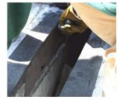
**WARNING** – Epoxy will harden more quickly when left in the pot. Apply it onto the joint faces as soon as possible.
