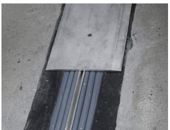
The SJS System installed with Emcrete elastomeric nosing material in blockouts on each side of joint gap.
