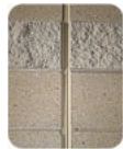
An expansion joint set in place that maintains the performance properties of the interior wall system. The watertight silicone outer seal of the precompressed, impregnated foam joint is manufactured to color coordinate with the tile and stone façade of the wall.
