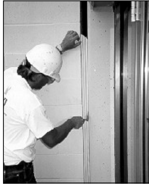
Figure 5: Hybrid silicone/impregnated foam sealant is inserted into joint-gap.
